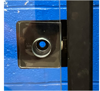
Clamps fasten through glass to prevent separation or slippage.
